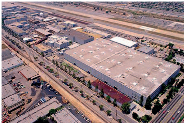
Aerial view of the new Hawthorne HQ of SpaceX, covering over 11 acres; Interior of the new building — just one “small” portion of it.
